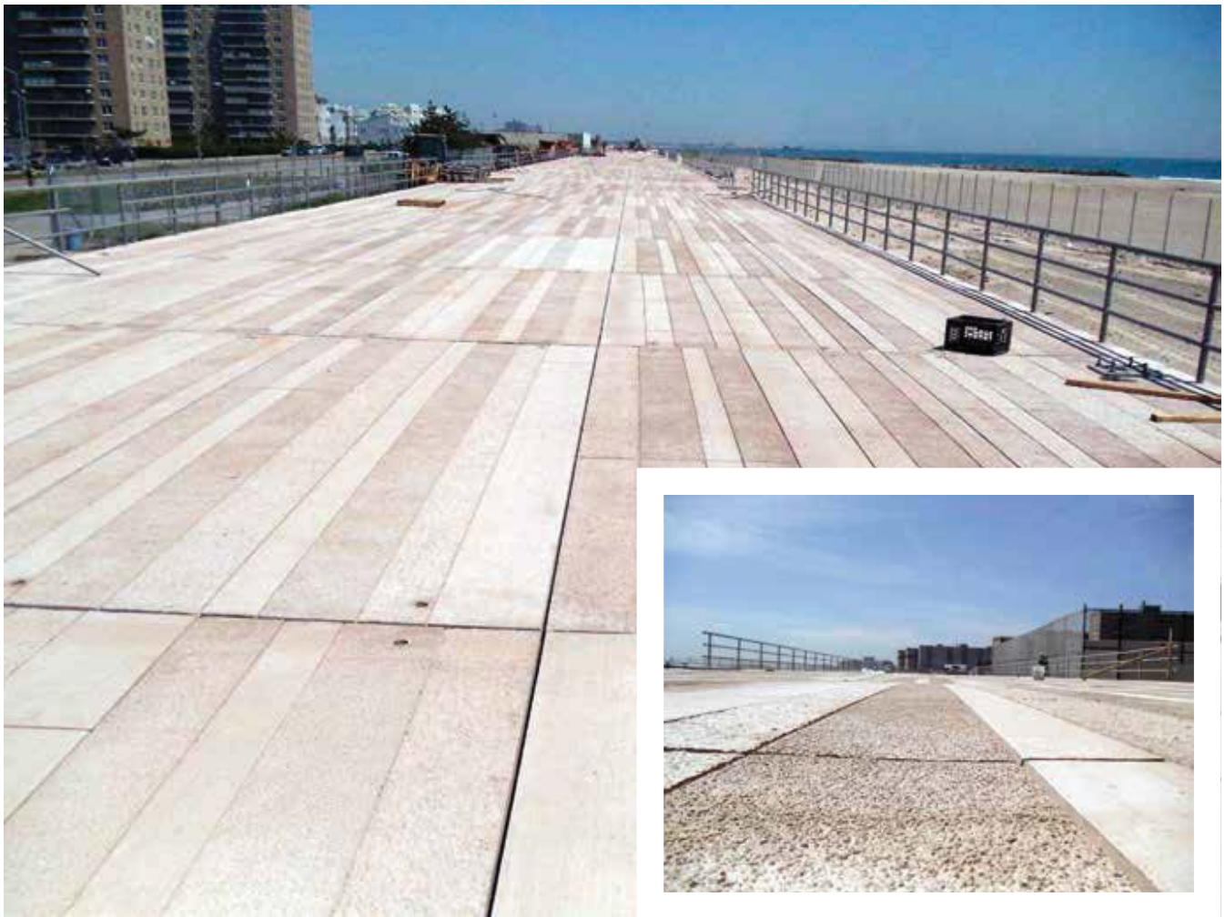
Precast concrete panels, formed to resemble five textured planks, were used in rows of five to produce an upgraded 10,000-linear-foot boardwalk in Queens, N.Y. The panels withstood Hurricane Sandy, the only portion of the boardwalk to remain intact. Photos: Steve Kenepf, U.S. Concrete Precast Group.
