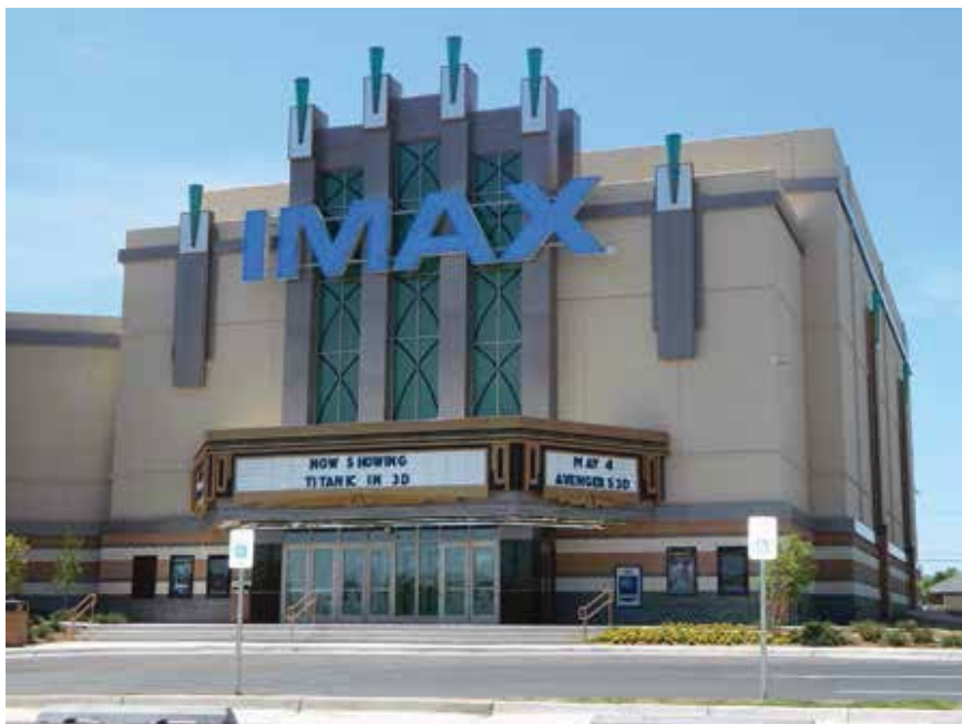
A number of factors allowed the precast concrete panels on the Imax Theater addition to the Warren Theater in Moore, Okla., to survive intact when tornadoes hit the area in May. Patrons survived without injury, and the theater was turned into an emergency center. Photos: Coreslab Structures (OKLA), Inc.
